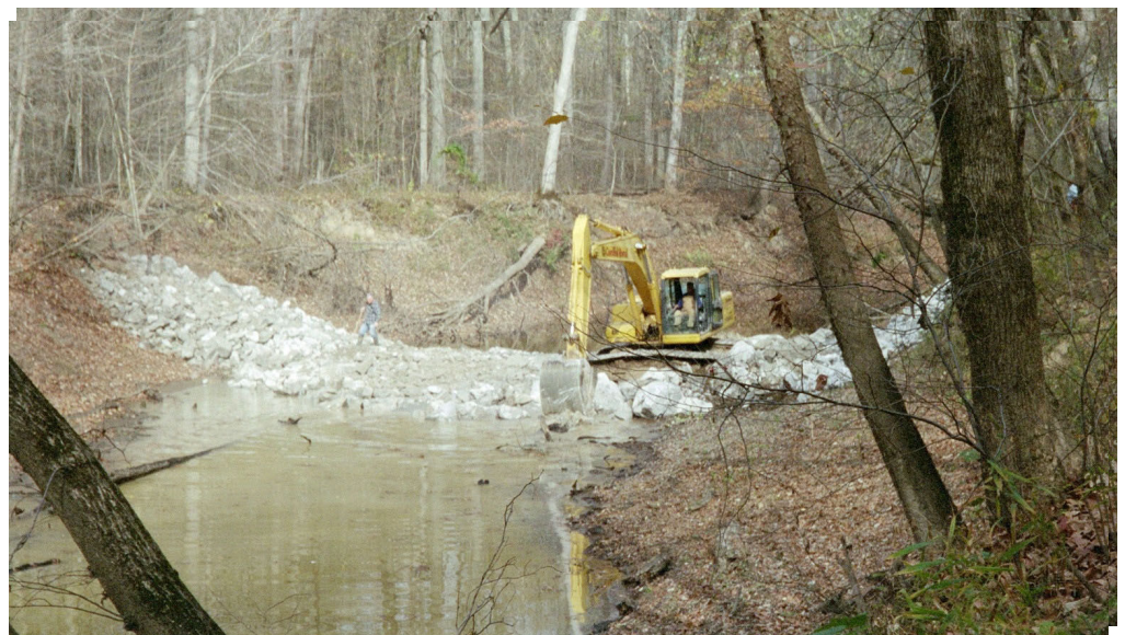
Figure 2. Newly constructed rock weir on the upper Cache River.
